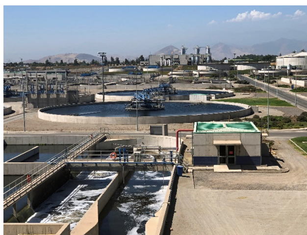
Santiago Waste treatment plant Source: 4D Infrastructure
