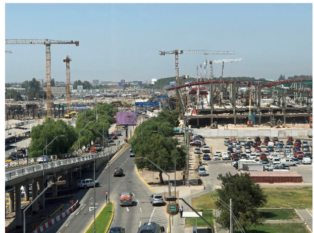
Santiago airport construction Source: 4D Infrastructure
